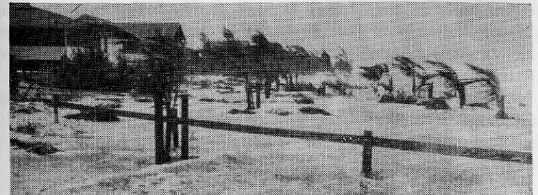
Just south of Red Coconut Trailer Park during 1926 hurricane.
